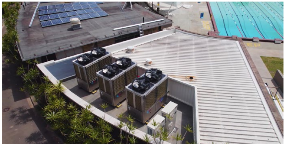
Electric heat pumps replacing gas at Victoria Park Pool. Credit: Supplied by Image Air
